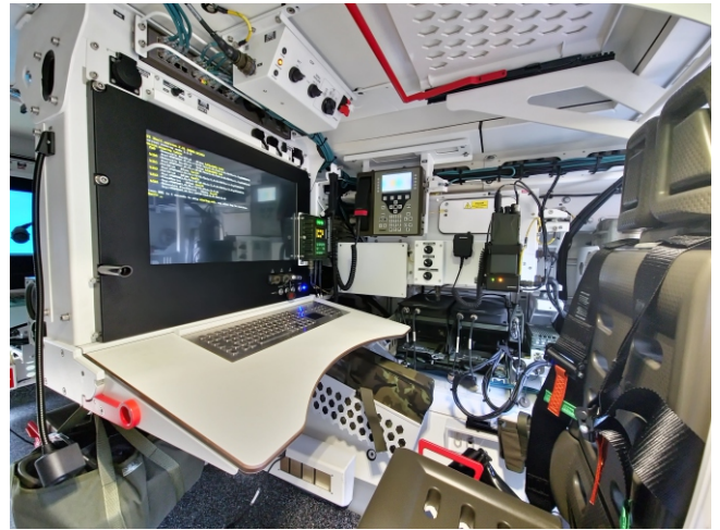
OPTOKON ruggedized phone LMIPT installed in TITUS
